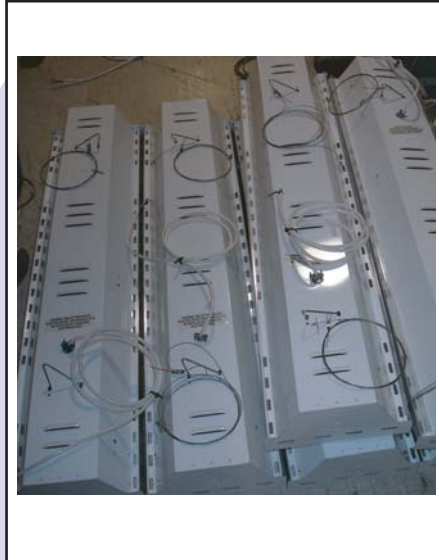
Pre-Installed hangers on fixtures
